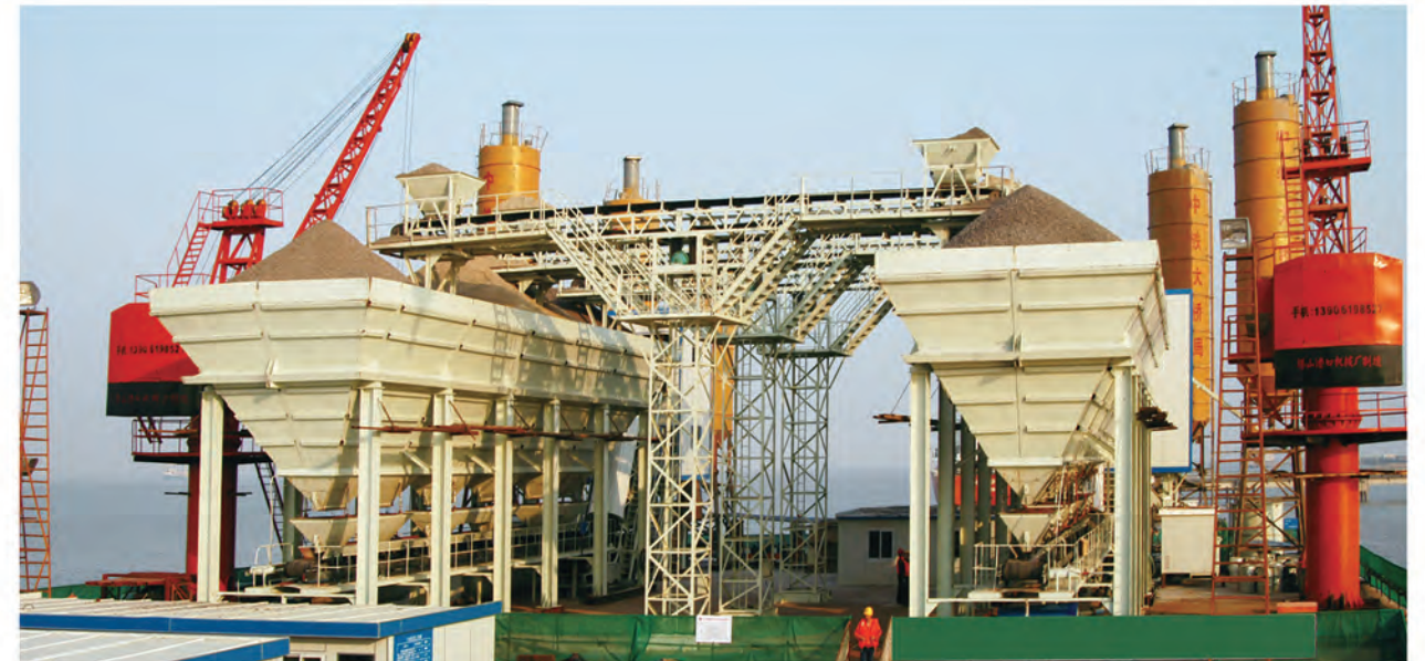
▲ Mixing plant on water platform
